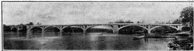
Section of Apalachicola River Bridge, Florida, during construction. Total length 5500 ft.
